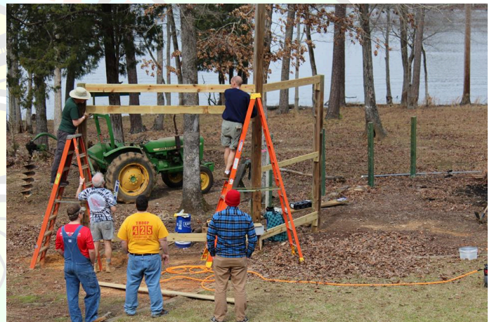
Campfire Area upgrades underway
