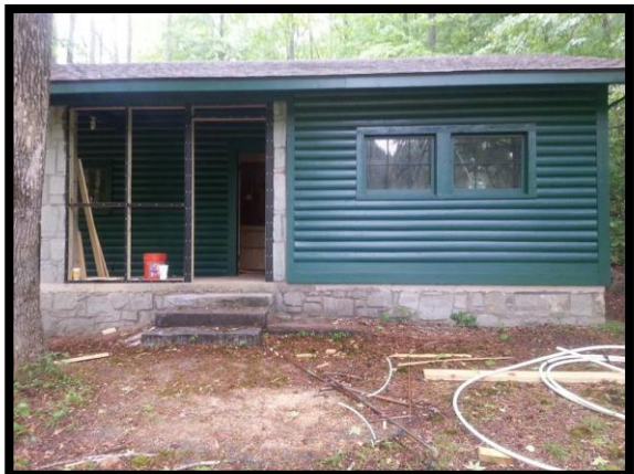
DC Cabin Renovation Project - 2015
