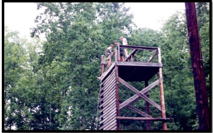
Old COI Climbing Tower - 2000
